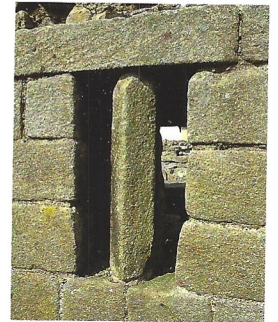
Below: The only surviving mullion in a granary ventilator slot in Britain is in the east granary at Corbridge
