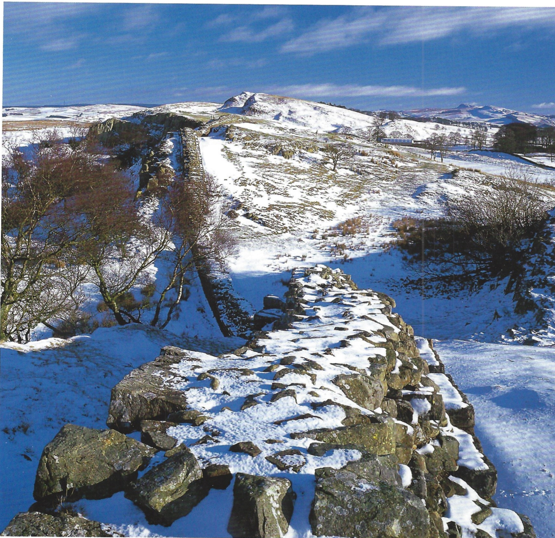
Left: Hadrian's Wall at Walltown Crags, in the central sector
