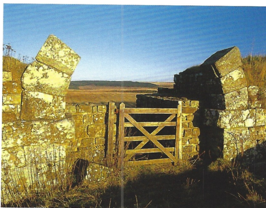
Left: The north gate of Housesteads milecastle. Some of the arch stones have been replaced
