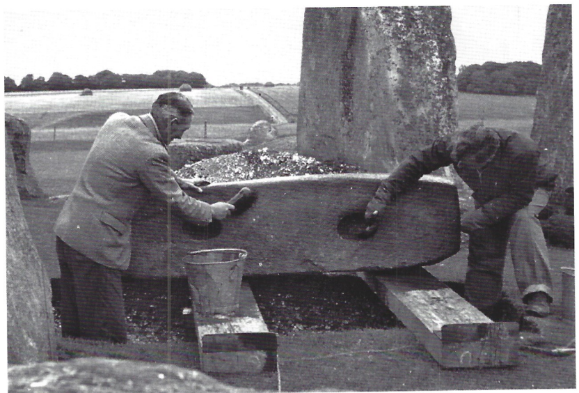
Below: A finely shaped bluestone lintel discovered during excavation in 1954
