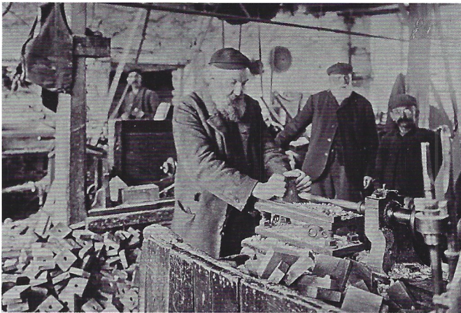
Left: Charles Jackson boring end pieces for bobbins on the upper floor of the old mill in about 1905. Originally indentured at Stott Park as an apprentice in 1839, he worked there for 68 years until he died in 1907
