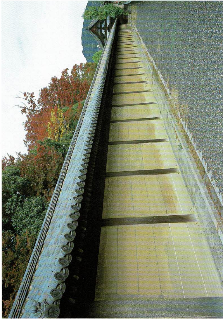
Taikou-bei : Earthen wall (Important cultural property : Momoyama period)
