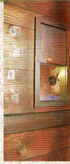
Fire watch window on the mezzanine floor Small window for watching out for fire in the irori fireplace
