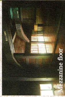
Fire watch window on the mezzanine floor Small window for watching out for fire in the irori fireplace
